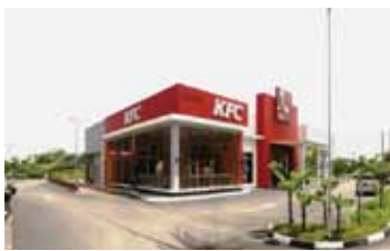
(A) Drive-through outlets
